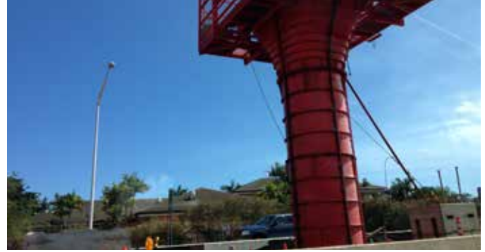
Fixed Guideway under construction in Waipahu
