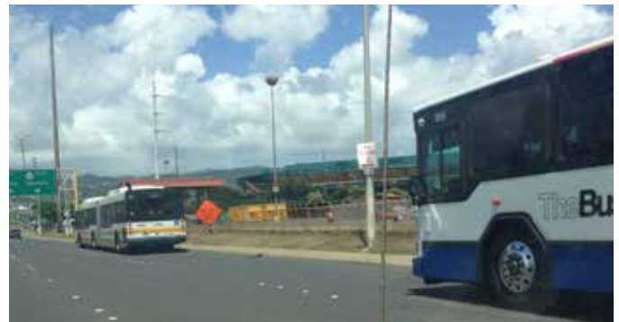
Future location of Aloha Stadium HRT Station
